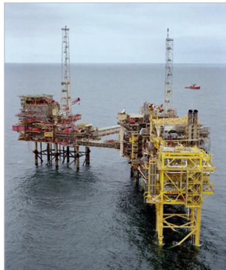
MultiSTEEL Project: Shell Clipper Platform (British North Sea)
